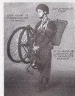
Fig. 1.—Airborne bicycle in jumping position
