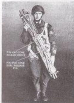
Fig. 5.—Airborne stretcher in jumping position
