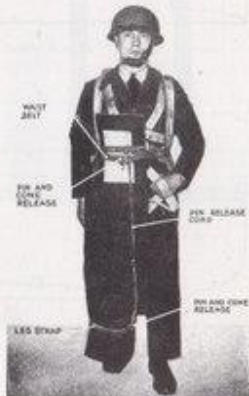
Fig. 6.—Bren gun valise Mk. II in jumping position
